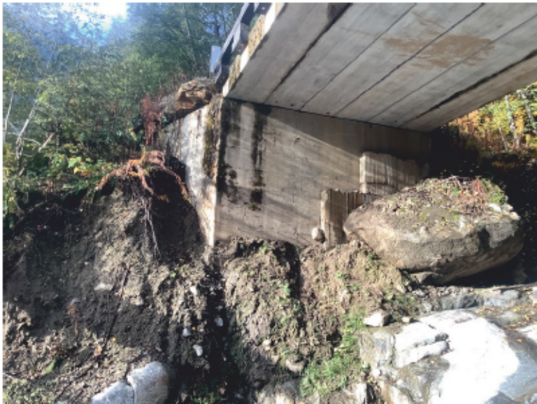
Right Bank Abutment when facing downstream
