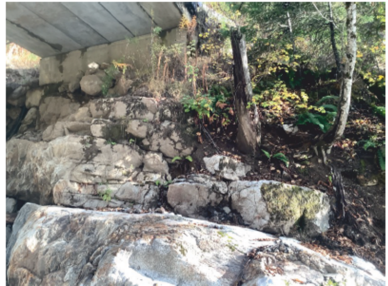
Left Bank Abutment when facing downstream
