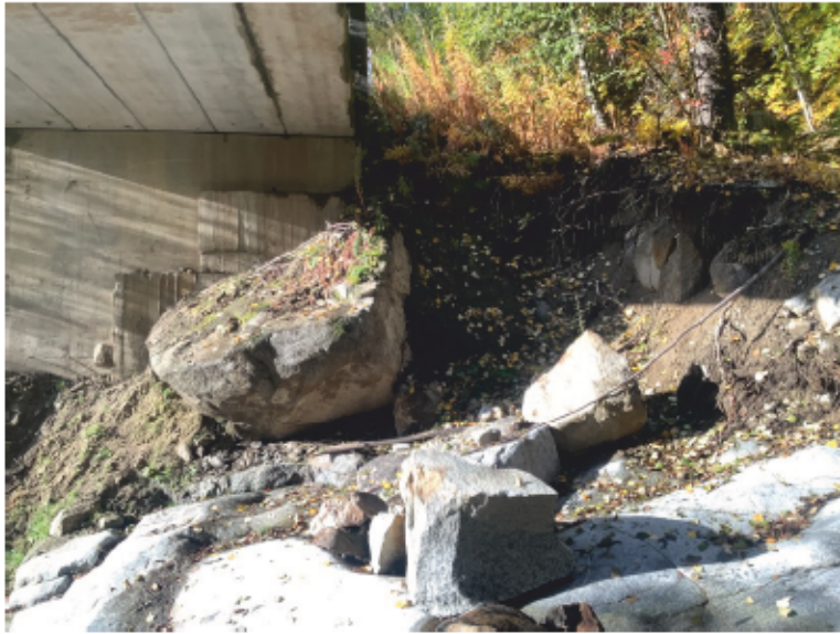
Right Bank Abutment when facing downstream
