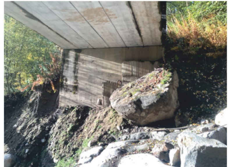
Right Bank Abutment when facing downstream
