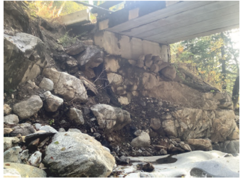
Left Bank Abutment when facing downstream
