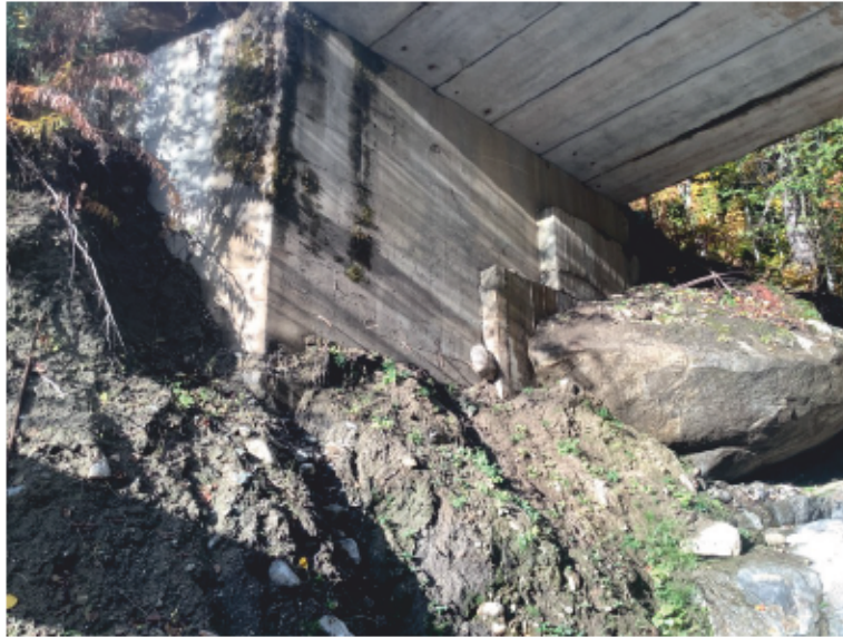
Right Bank Abutment when facing downstream
